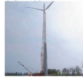
Henan 40MW Hybrid Tower Project
