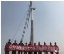
Henan 120m Hybrid Tower Project
