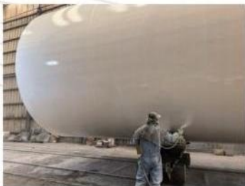
Beibutan Wind Power Project
