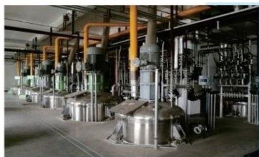
Topcoat Production Line
