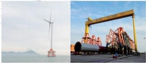
Zhuhai Guishan Offshore Wind Power Project
