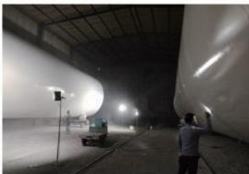
Ningxia Wind Power Project
