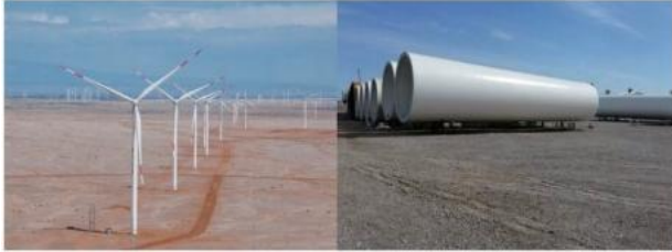
Xinjiang Wind Turbine Project
