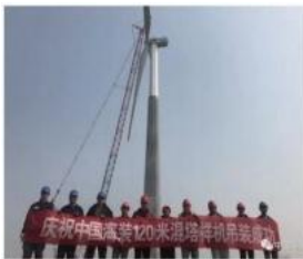
Henan 120m Hybrid Tower Project
