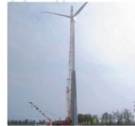
Henan 40MW Hybrid Tower Project
