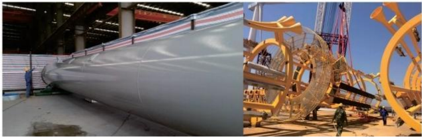
Three Gorges Xiangshui Offshore Wind Power Project
