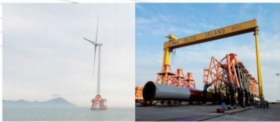
Zhuhai Guishan Offshore Wind Power Project
