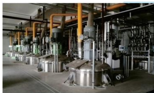
Topcoat Production Line
