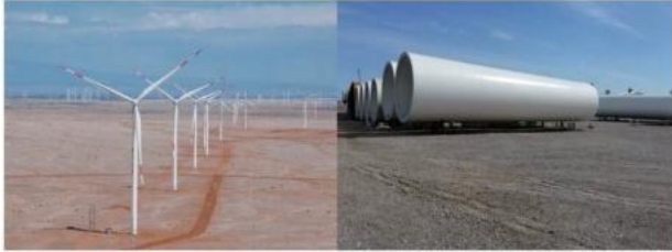
Xinjiang Wind Turbine Project
