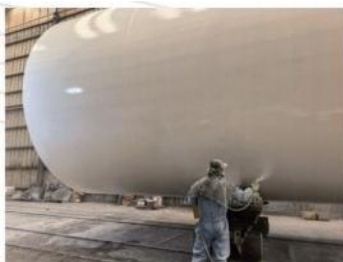
Beibutan Wind Power Project
